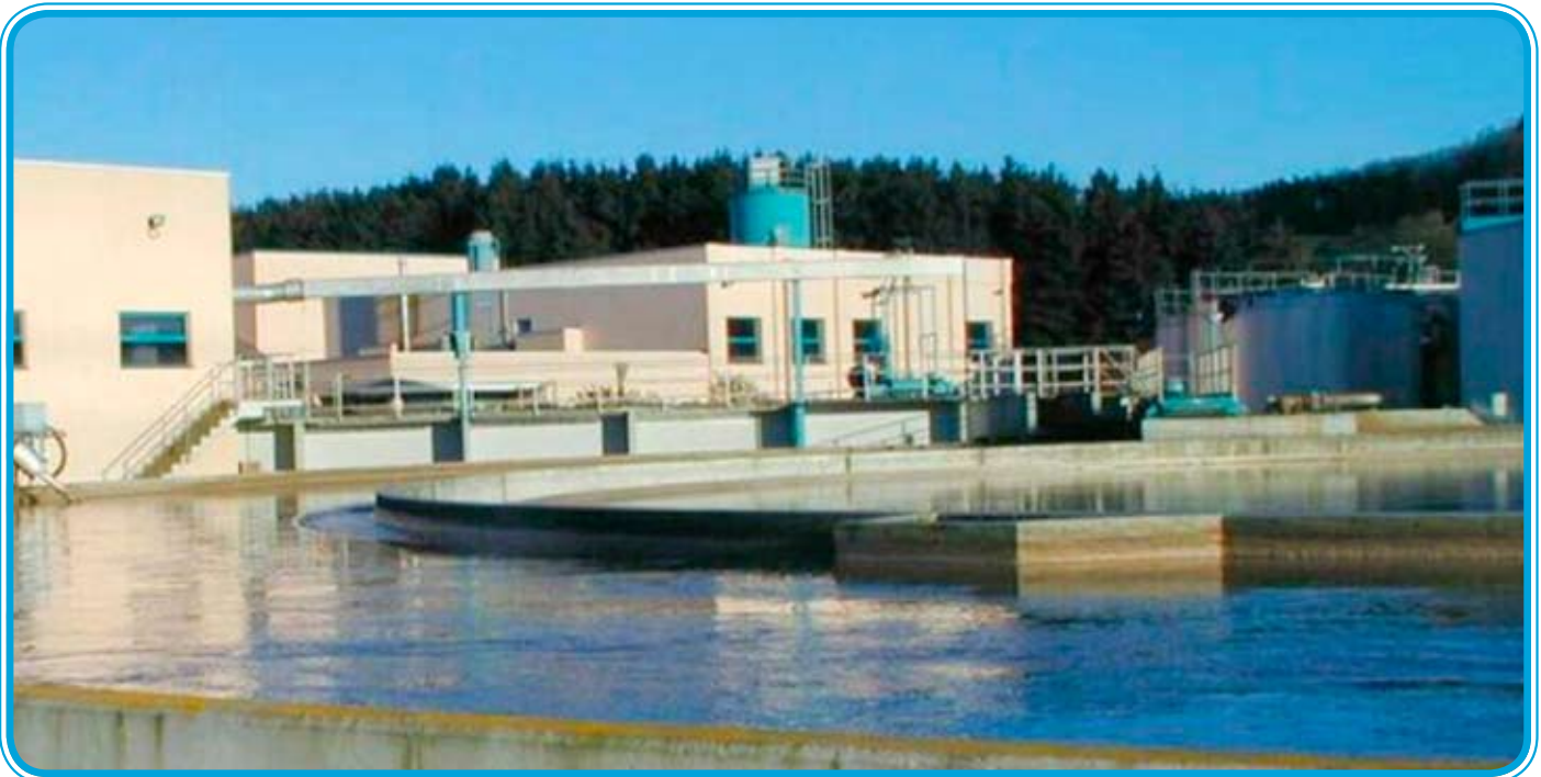
© Station d'épuration Uebersyren
